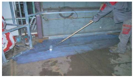
Spread out the DMS primer 54 smooth in a thin a layer at the floor Approx. 0,1 kg. / m<sup>2</sup>
