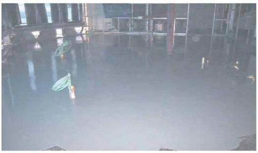
4. After app. 3-4 hours at 20°C. the floor is ready for walking and after 18-24 hours at 20°C and in a thickness of app. 8 mm. the floor is ready to be covered with carpet, PVC or tilling
