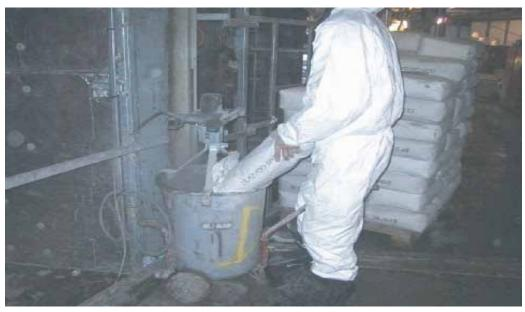
2. The measured quantity of water (4,5-5 liter) is added the mixer after this add the BH 3000 compound. Stir vigorously to a smooth, easy-flowing mortar
